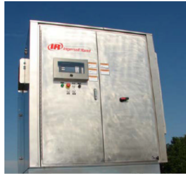
2 x MT250 (Offshore ): Thailand Stainless enclosure & C1/D2 Certified
